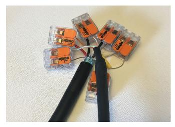
Figure 23 - DMX Termination Detail
